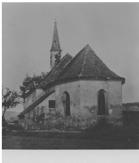
⬅ Fig. 2. View of the damaged church of St. Jošt in Cheb (photoarchive of National Heritage Institute, Directorate-General, Nr. N090456)
