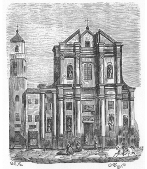
⬆ Fig. 6. Historic image of the Church of St. Martin, Warsaw (archive of author)
