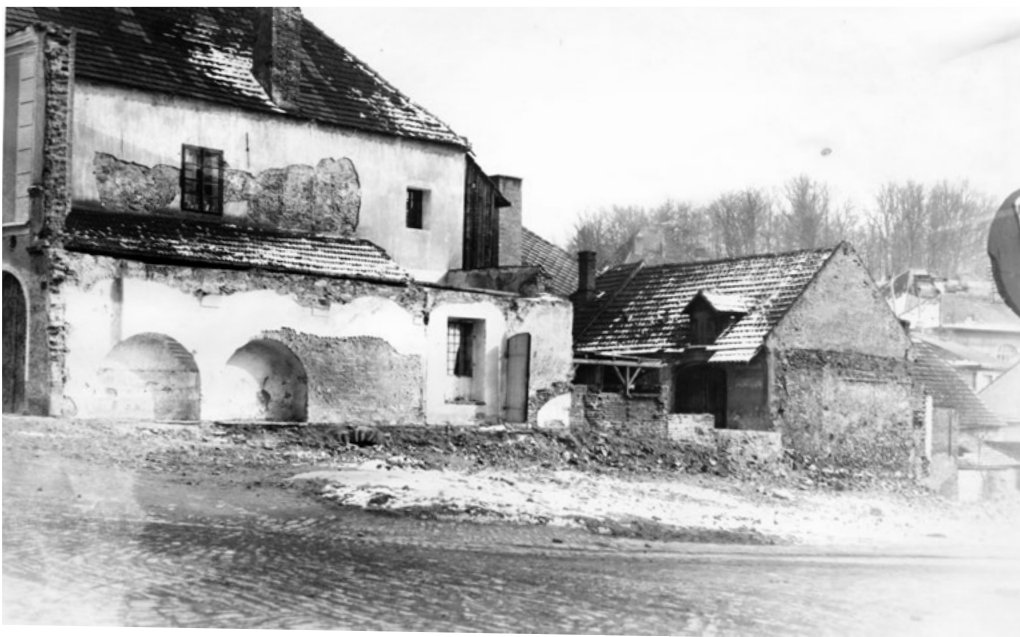
⬆ Fig. 10. Týn nad Vltavou, demolition of townhouses within reach of the rising river level, 1962 (Photoarchive of the National Heritage Institute, Regional Office in České Budějovice)
